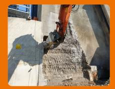
Removing concrete from the central pier. The upper section remained untouched while a 1.6 m deep layer was removed from the lower section.
