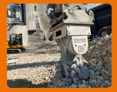
The KEMROC KR 120 in close-up. While working in unreinforced concrete, wear on the picks was minimal.
