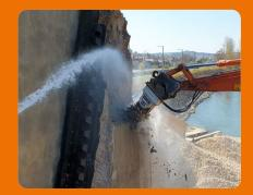
A KEMROC drum cutter working on the river barrage at Viereth on the Main. During renovation, the shape of the concrete pillars had to be changed.
