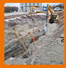
A sub-section of the A3 autobahn upgrade project in northern Bavaria. Drainage pipe trenches were excavated on site at the Steigerwald service area.
