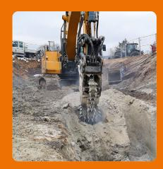
Civil engineering company BUNTE rented a 42-ton excavator with a KEMROC EK 150 chain cutter to excavate trenches in the bedrock.
