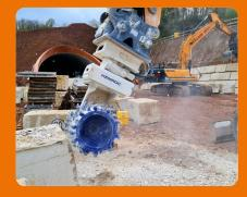
The new A44 autobahn from Kassel to Herleshausen is taking shape. At the eastern portal of the new Trimberg Tunnel, a KEMROC ES 60 HD universal cutter on a wheeled excavator is playing a role.
