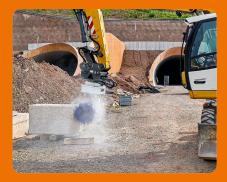
As the KEMROC cutter has been working well at the eastern portal, another machine of the same type has been delivered to the western portal of the tunnel.
