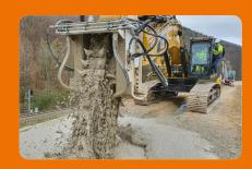
The cutter chain penetrates into the ground and mixes it with a binder suspension fluid from a semi-mobile mixing plant. After hardening, a homogenous, dense, load bearing soil-cement structure is created.
