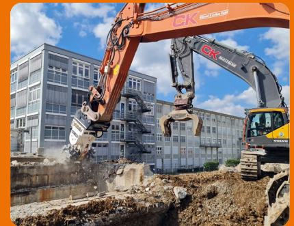
Drum cutter attachments used near buildings on the boundary. Unlike cutter wheels, they can work right up to the boundary.
