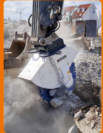
KEMROC cutter wheels with powerful motors and narrow cutter wheels play a central role in environmentally friendly demolition.
