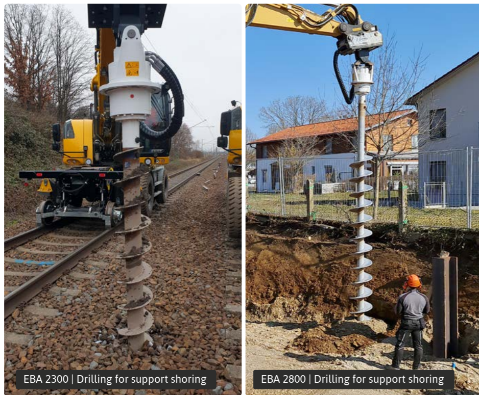
EBA 2300 | Special foundation work
